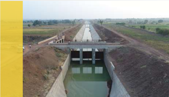
HEAD REGULATOR AND LINING OF MWC 0 TO 10KM
